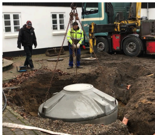
BioKube Betong installeras
