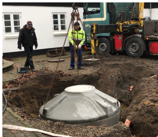
Biokube betong under installation
