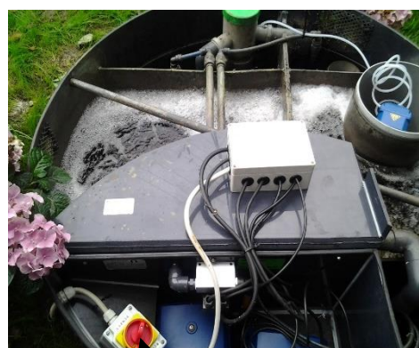
Power supply to BioKube
