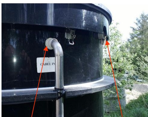
Cable inlet for technical box
